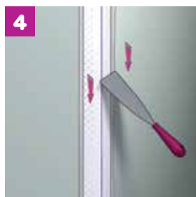
4 To remove excess compound and air bubbles, use a spatula
