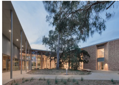
BERNINNEIT CULTURAL AND COMMUNITY CENTRE JACKSON CLEMENTS BURROWS ARCHITECTS
