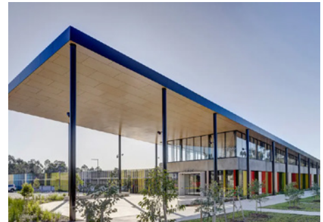
BLACKTOWN ANIMAL REHOMING CENTRE (BARC) SAM CRAWFORD ARCHITECTS
