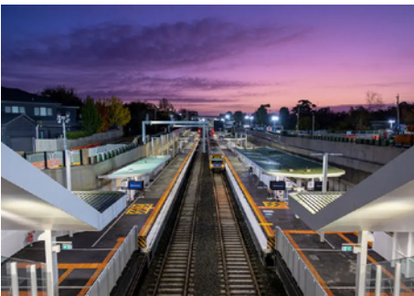
UNION AND MONT ALBERT LEVEL CROSSING REMOVAL PROJECT – UNION STATION SOUTH EASTERN PROGRAM ALLIANCE
